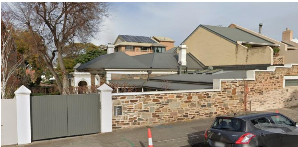
Figure 13: 112 Brougham Place Sandstone fencing with late, Streetview, July 2020
