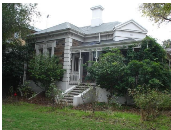
Figure 14: South elevation of 112 Brougham Place (rear facing, away from the street). Source: CoA
