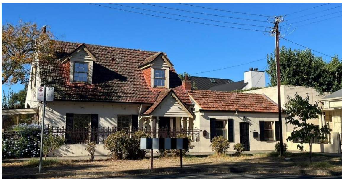
Figure 17: 39-40 Kingston Terrace. Source: Google Street View
