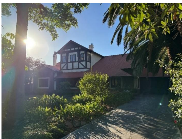
Figure 27: 424 Gilles Street with garage addition, CoA
